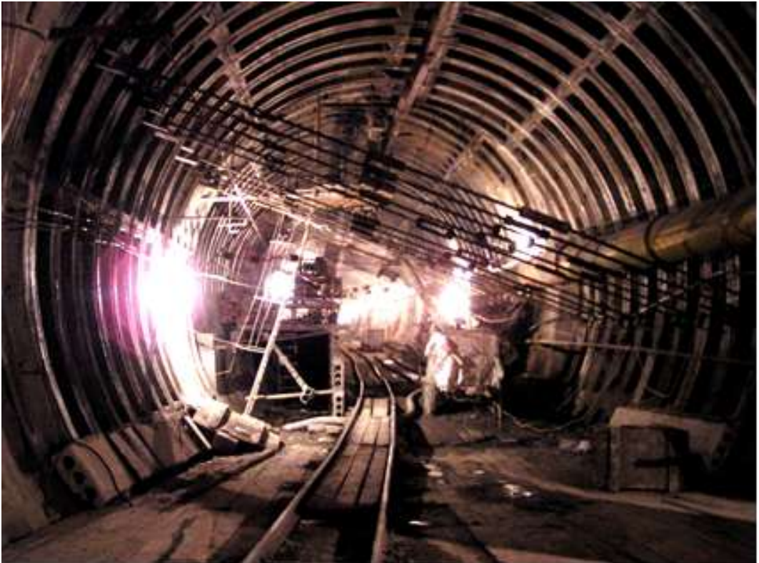
Fig. 2. Measures to restore geometry of transport tunnel processing
