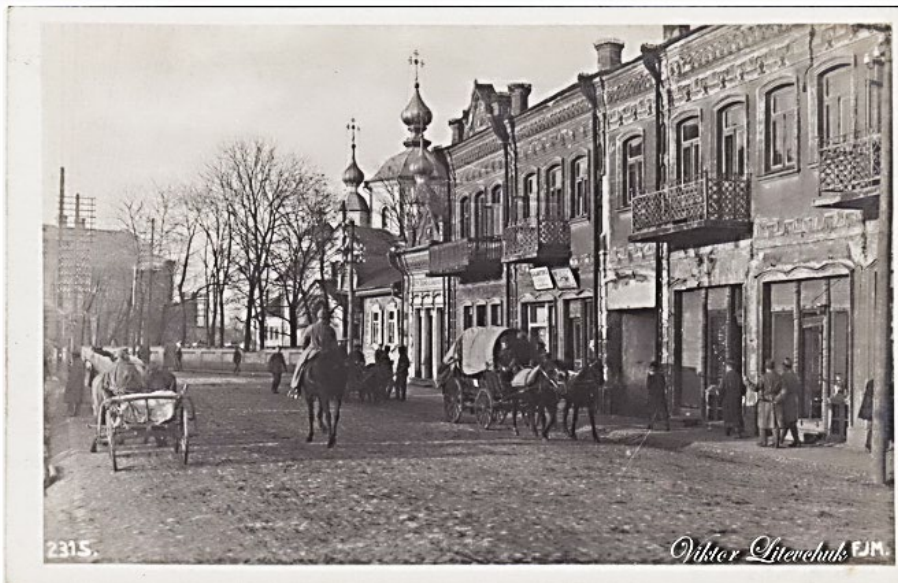
Fig. 5. Lutsk street in Kovel. Karl Harbauer's publishing house, Vienna, 1916
